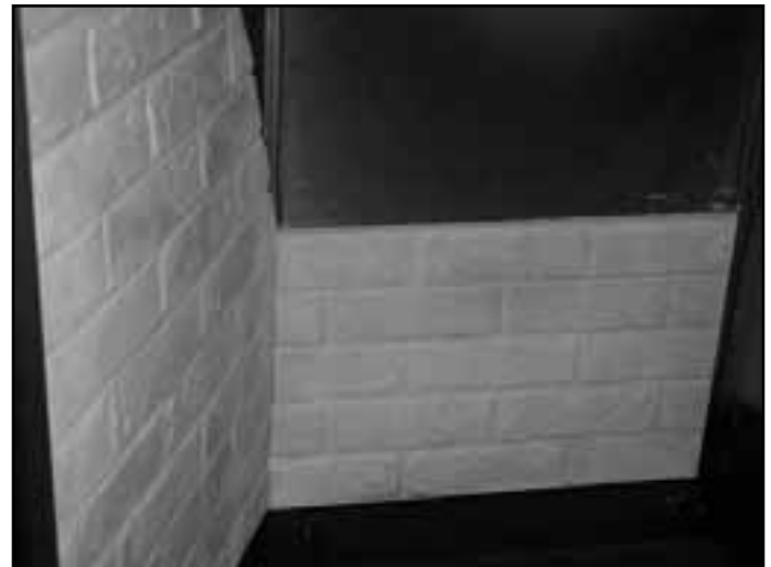
Figure 14.3 Install Lower Back Refractory
